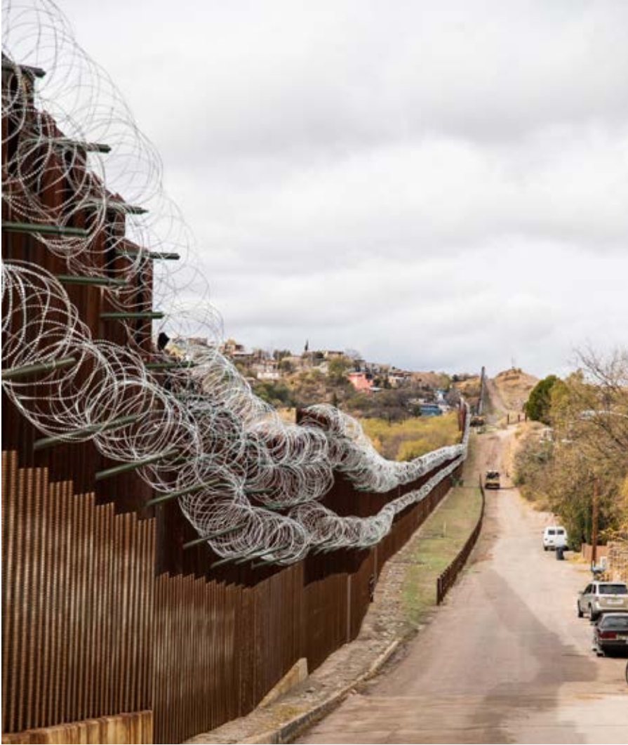
KEEP OUT: Layers of Concertina wire are added to existing barrier infrastructure along the US-Mexico border near Nogales, Arizona
