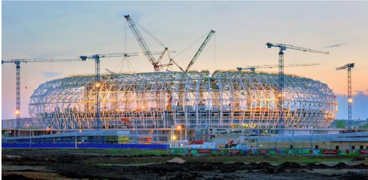
Work on a new stadium in Saransk for the 2018 World Cup.
