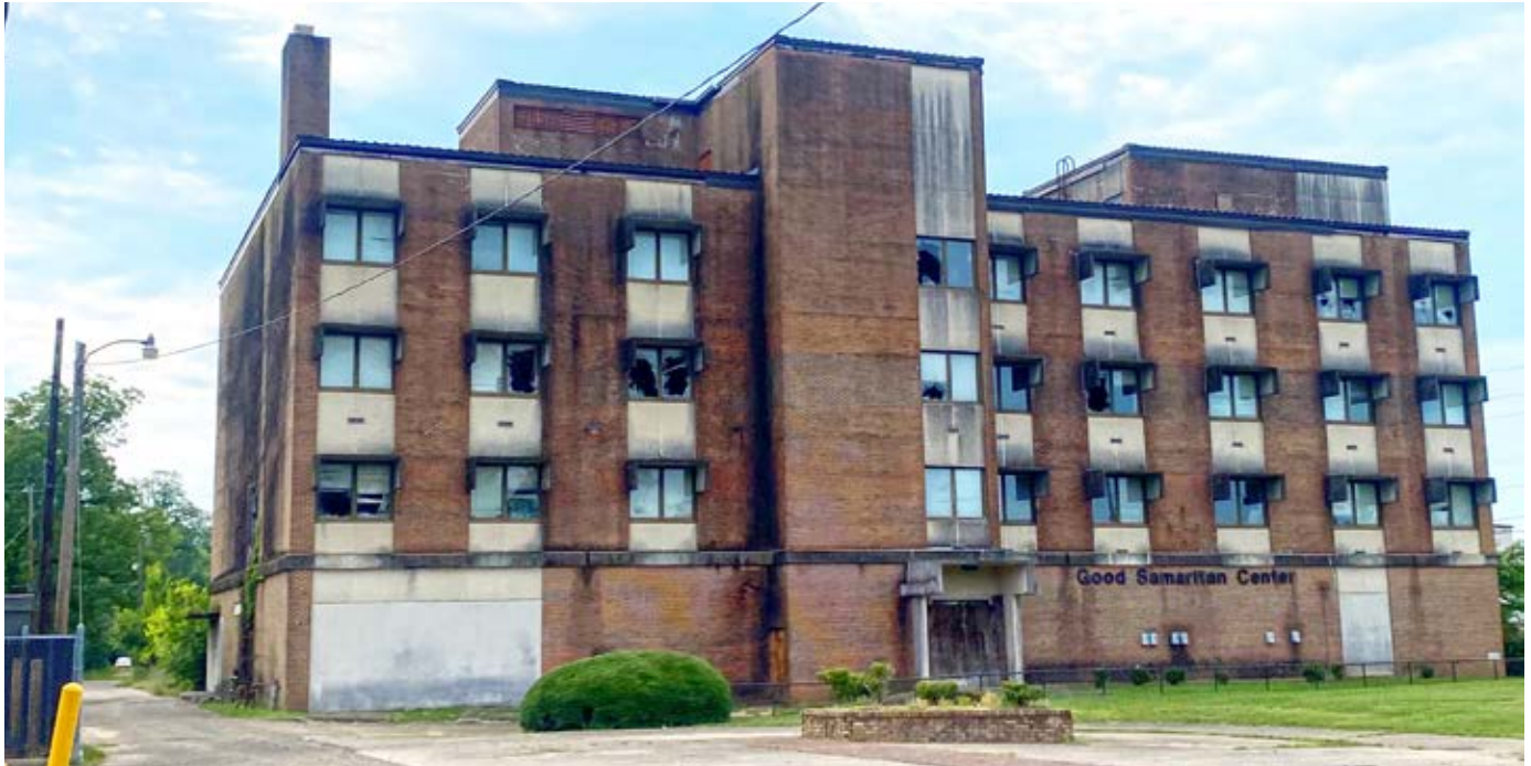
The boarded-up Good Samaritan Center apartment block
