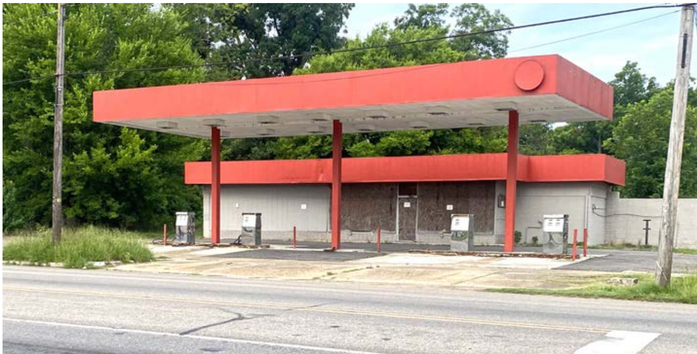
An abandoned gas station on Broad Street, Selma.
