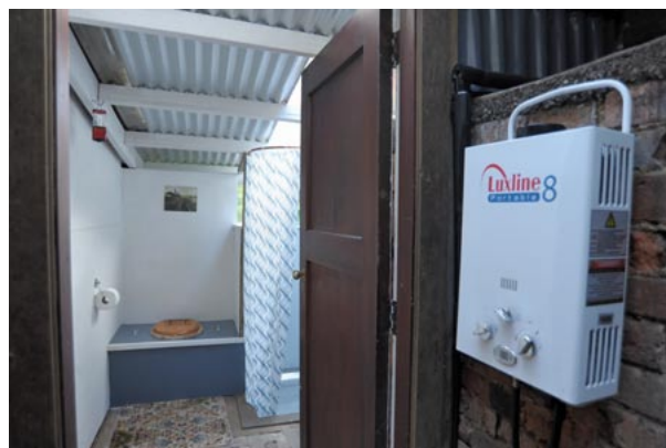
AFTER: Indoor 'composting' toilet, shower and gas heater.
