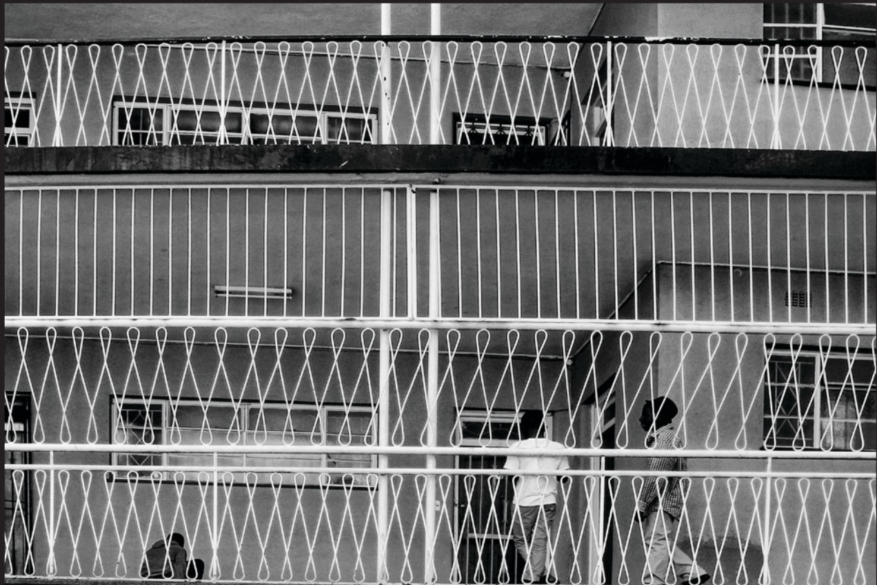
No, not a prison, it's an apartment block in Rosebank, Johannesburg. Now that the country has moved from apartheid to 'equality', fear has no colour: middle class blacks are as afraid of the underprivileged as are their white neighbours.
