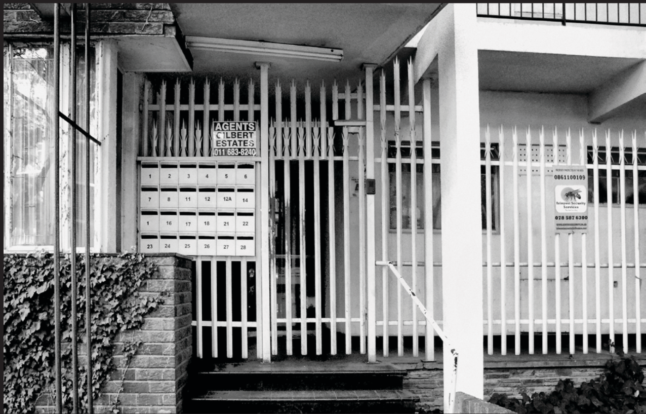
Rosebank, Johannesburg - It's not just the rich who are afraid of being robbed by their poorer cousins; working class apartments are surrounded by railings and protected by gun-toting security contractors. And the bars and locked doors look, to an outsider, like self-imposed prisons.
